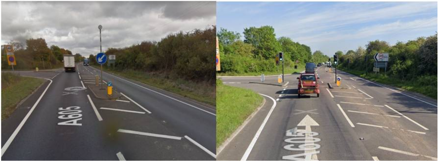
Figure 2: A605 Before and After Signal Installation
